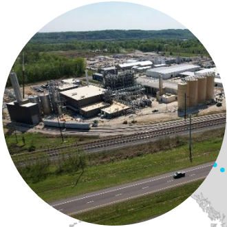
IRONTON, OHIO PREP, PURIFICATION & COMPOUNDING FACILITY
