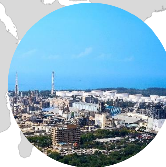
RAYONG, THAILAND FUTURE PURIFICATION FACILITY
